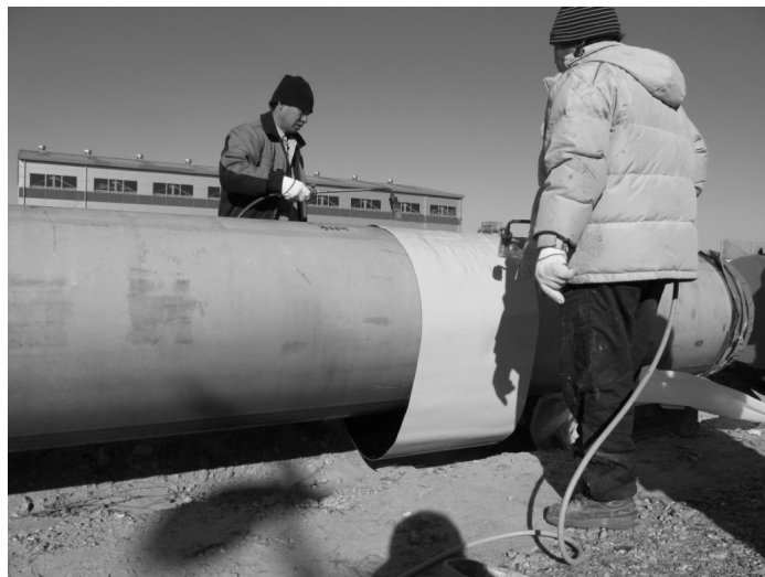
Figure 9. Coating Application for Field Test of Coating Performance
