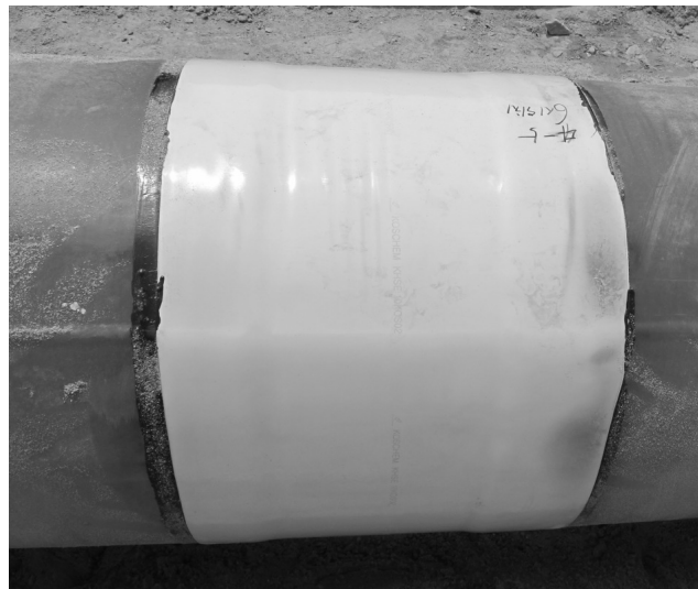
Figure 11. Small Wrinkles on the Surface of Excavated Buried Pipe (C group-5)
