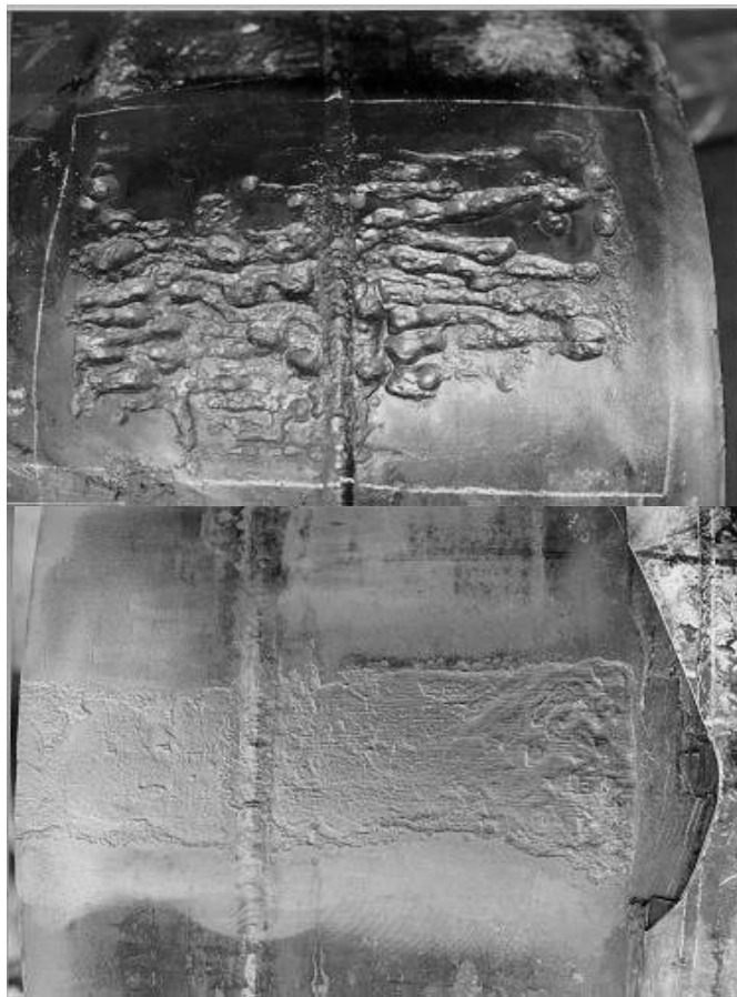
Figure 3. Corrosion of Pipe at the field applied coating failure
