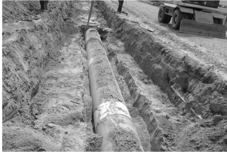
Figure 10. Excavation of the Buried Pipe for Field Test of Coating Performance
